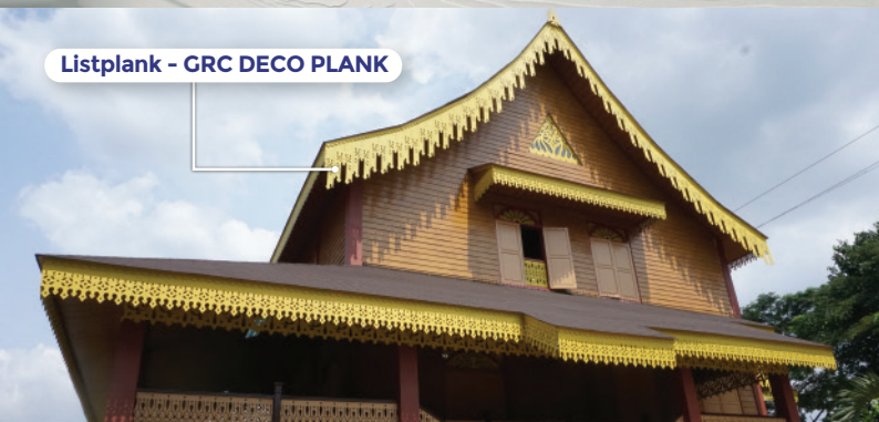
Fasad - GRC ROSEWOOD PLANK
