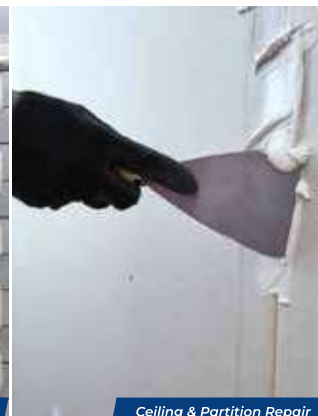
Ceiling & Partition Repair
